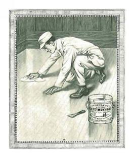
Laying the foundation for the finish by filling the pores with Wheeler's Paste Wood Filler.
