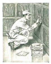
After thinning Wheeler's Paste Wood Filler, apply it to the surface of the wood with a brush, allow it to set five or ten minutes, then rub well into the porce of the wood with a cloth and wipe off the work thoroughly.
