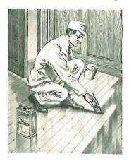
Applying Bridgeport Standard Floor Varnish Over a Foundation of Wheeler's Paste Wood Filler.
