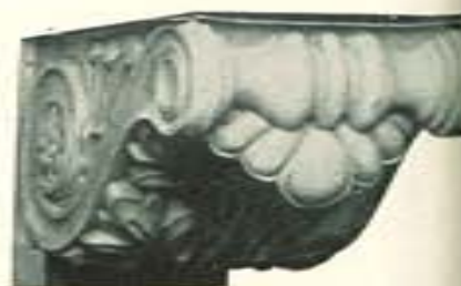
No. 7171. Pro., 19¼ in.; depth, 11 in.; face, 12 in.; in parts, each, $8.50.
